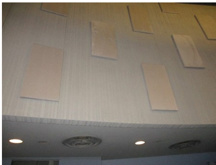
Figure 3: Sound proofing panels found on the walls of an auditorium.
